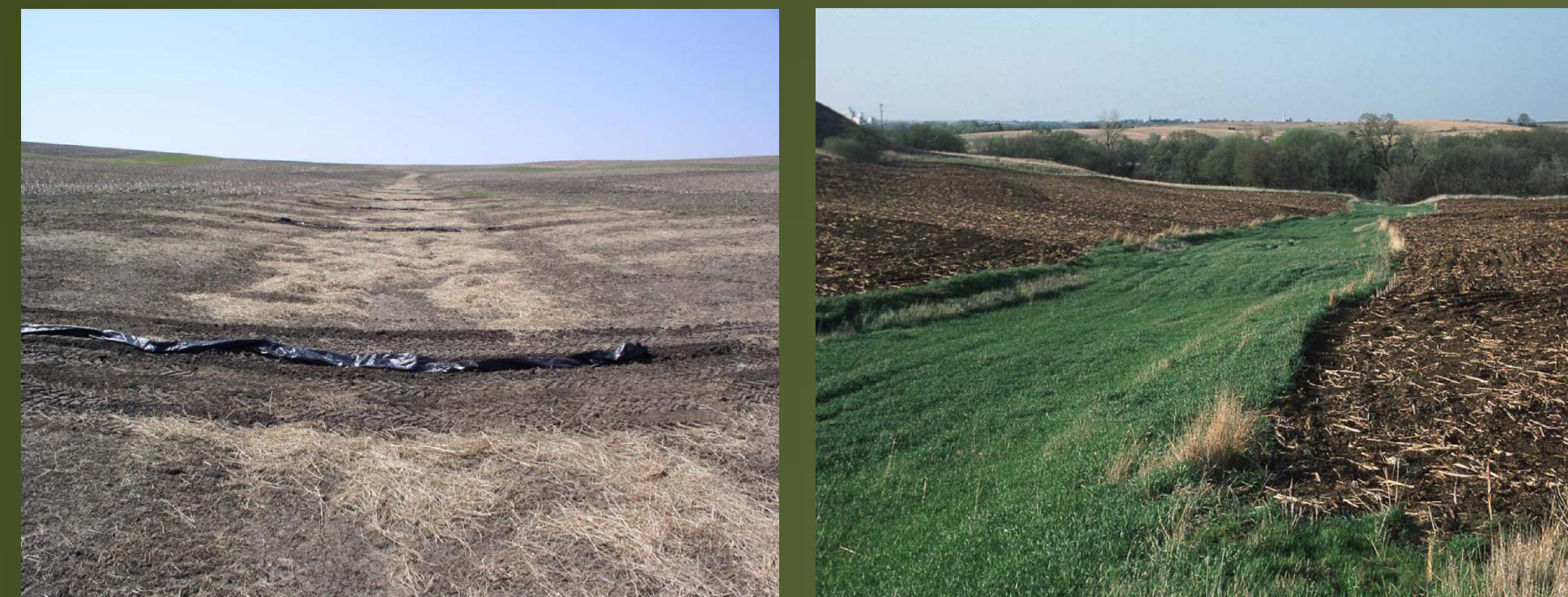
Construction of the GWWs in eastern Iowa
